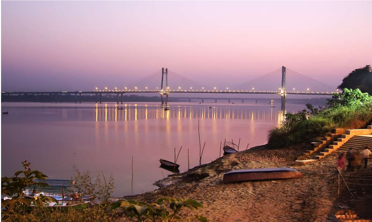
Bridge over river Yamuna at Allahabad
