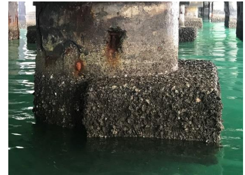
Concrete immersed in sea water
