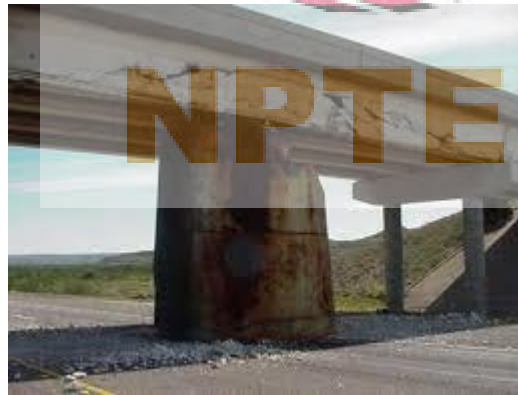
Cracking/disintegration
