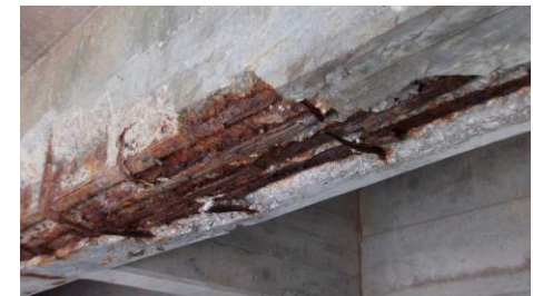
Corroded/exposed rebars
